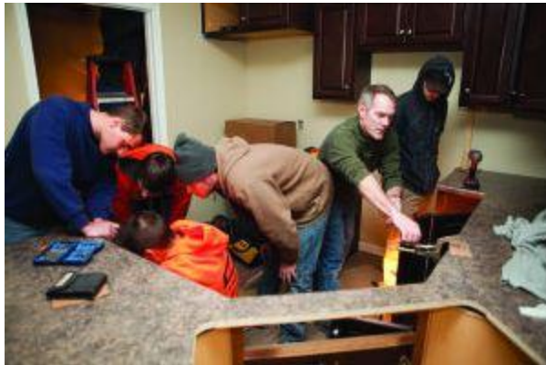
Iowa Western Community College Construction Technology Instructor Rob Klepfer, center, works with Allen Murray, right, while Dusty Winchester, far left, inspects cabinets and drawers with fellow students at a project house March 27.
